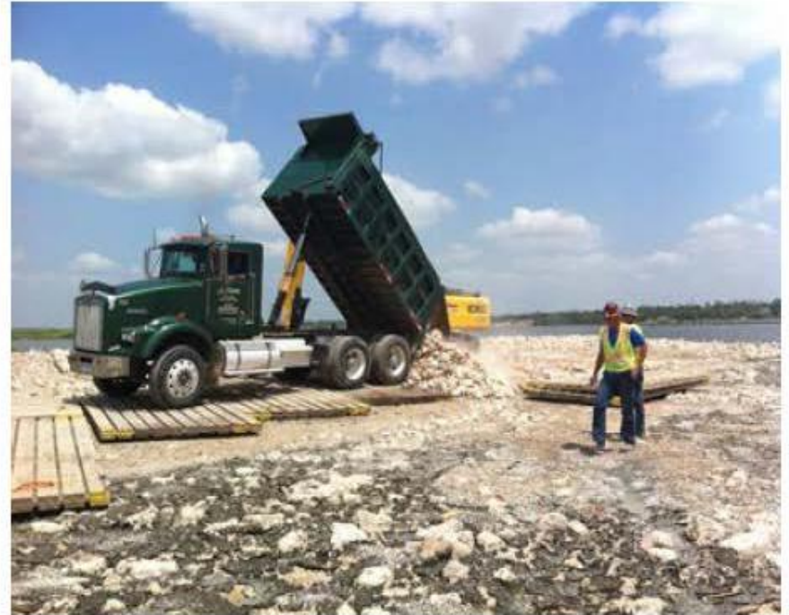
Dump truck off loading rock for placement
