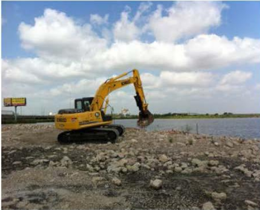
Cap repair with trackhoe placing rock over area with erosion
